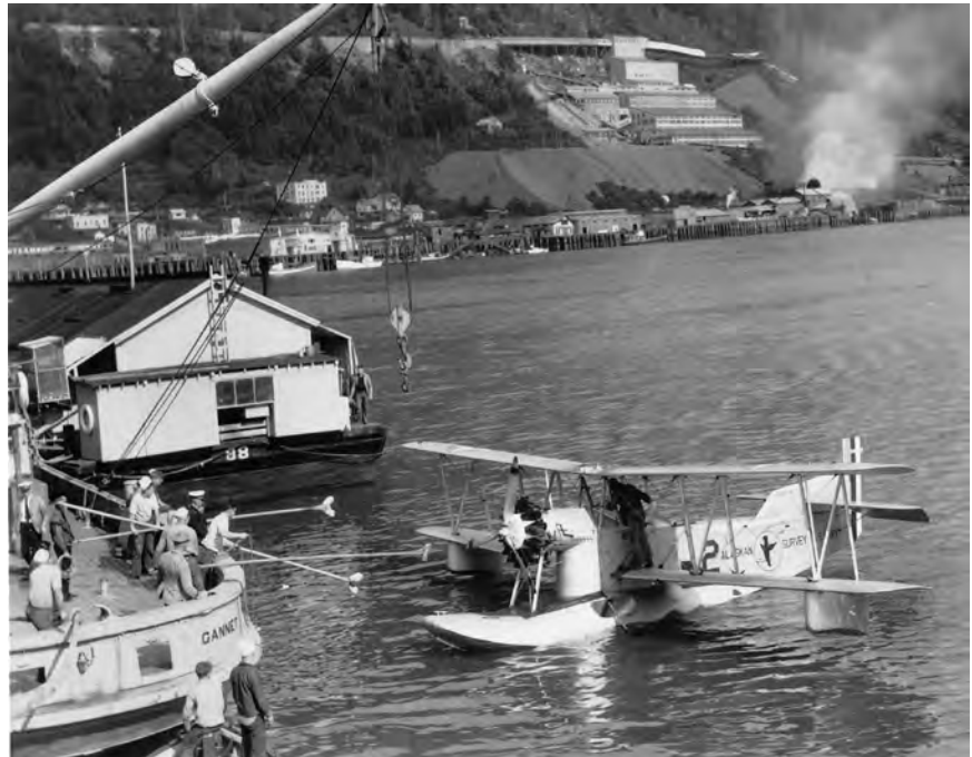
Figure 28. —1926 photograph of Alaska Aerial Survey Expedition operations in Juneau Harbor, showing the stern of the tender Gannet; one of the open-cockpit Loening Amphibian biplanes used to obtain aerial photography; and the stern of the 140-ft-long barge used for photographic and film-processing operations. Photograph Alaska 363 from the USGS Photographic Library, Denver, Colo.
